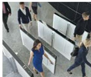
Direct home floor call feature can be activated when Destination Control System and turnstiles are integrated.
