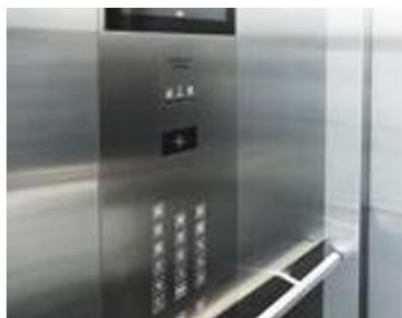
Card reader in Car Operating Panel (COP)
